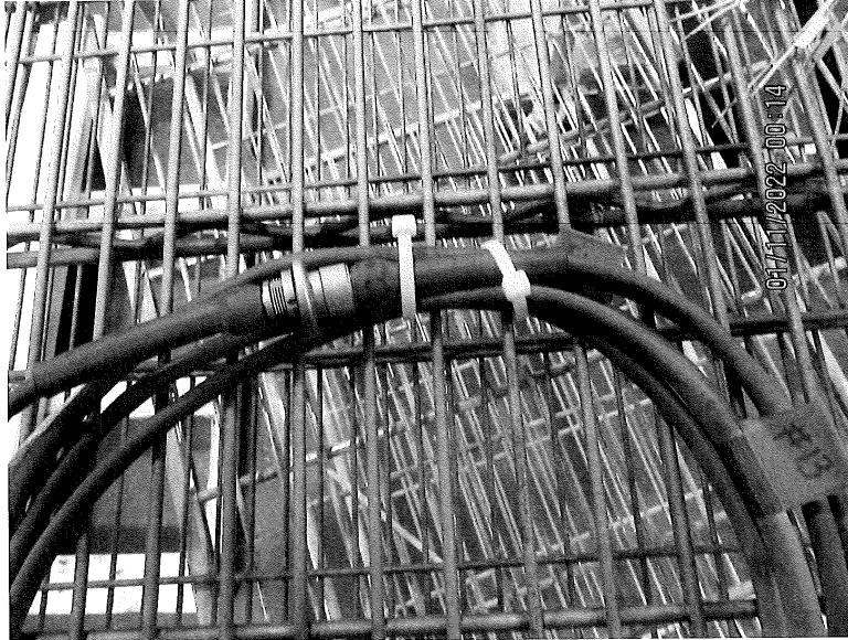
Photo 1 – File No. 0622-0011 Post-test photo Set 1
